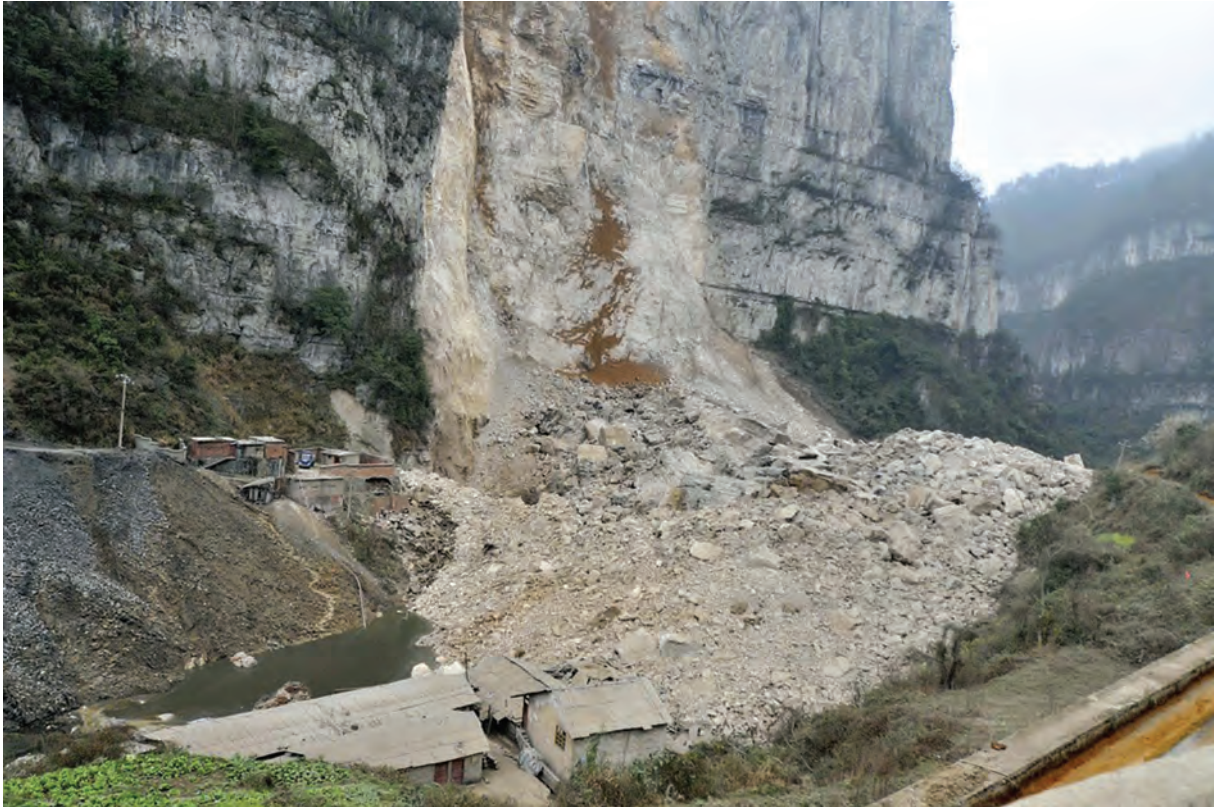
A large rock fall
