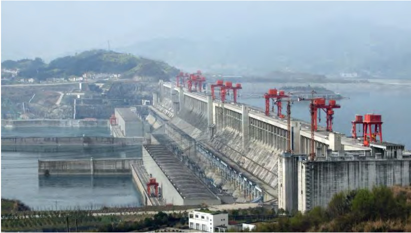
Fig. 1 – The Three Gorges Dam, China
